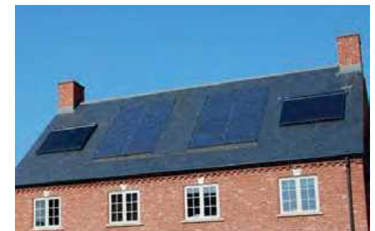
Solar panels reduce energy demand and lower running costs but need to face close to south and lie at 45° for maximum efficiency.
