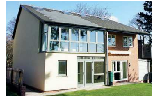
A large window for solar gain and a deep overhang and canopy for shade.
