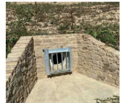
Stone clad headwalls.
